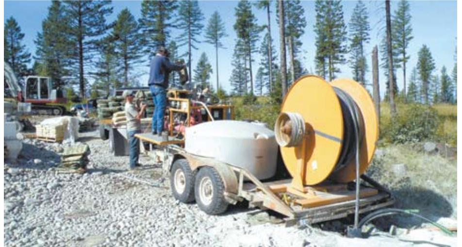
Keep in mind that thermally enhanced grout produces the desired thermal conductivity in the borehole to accommodate the GSHP system, and helps to prevent the co-mingling of any aquifers encountered in the borehole.
