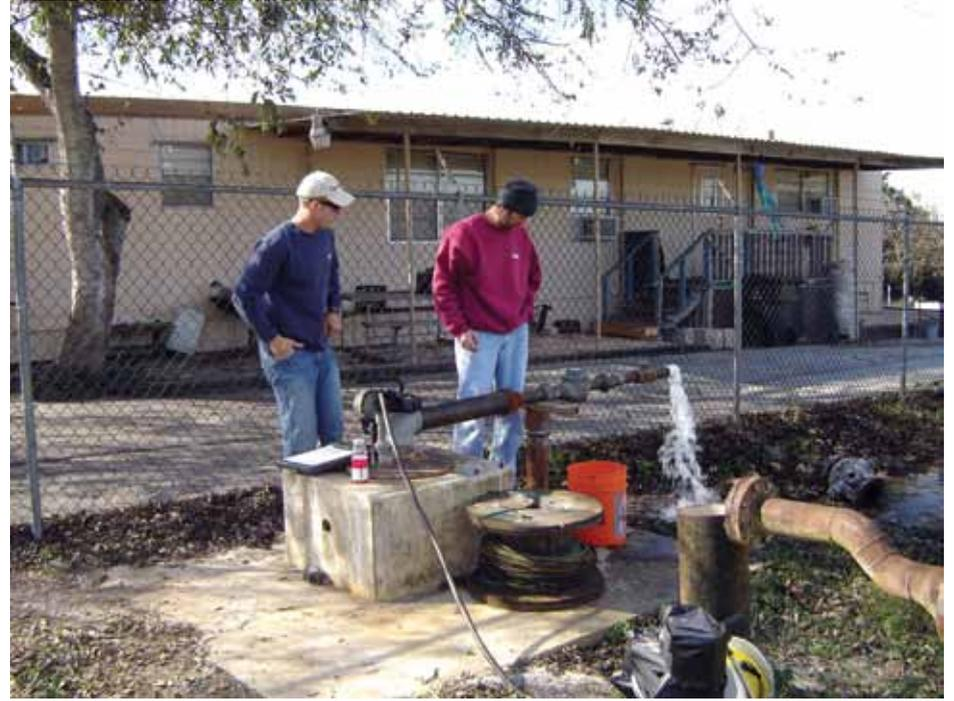
Mechanical cleaning also is necessary to ensure success. Running a pumping test after completing well rehabilitation. Photo courtesy of Kyle Murray, Ph.D.
