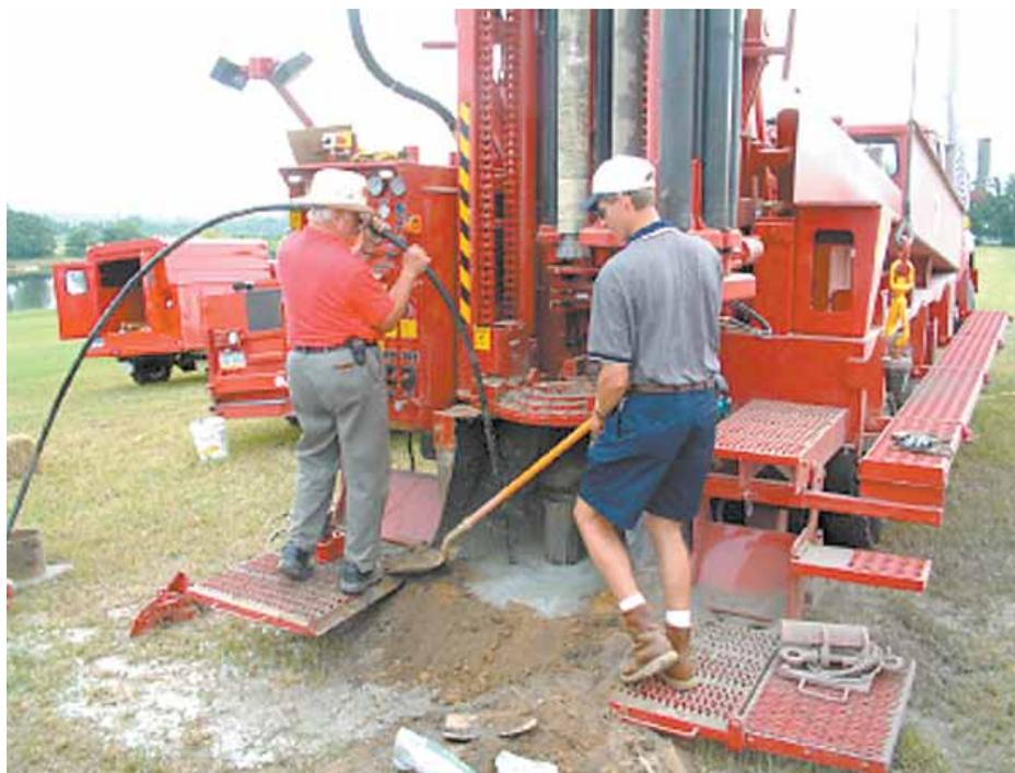
Using a tremie pipe to place bentonite grout into an annular space. Photo courtesy of the Pennsylvania Ground Water Association.
