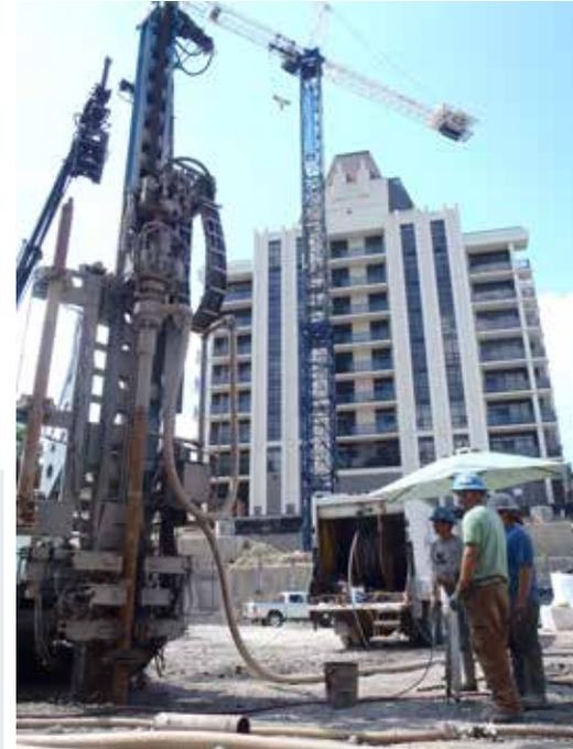
Oakville Hydro Energy Services commissioned Geosource Energy Inc. to install geothermal heat loops for a new condominium complex being constructed by an Ontario developer, Ninco Construction Ltd. The building, called the Roman, will be a 6 story multi-residential building that will be approximately 40,000 square feet.
